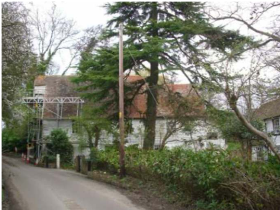
Fig. 21. The Grade II* listed Spring Valley Mill
